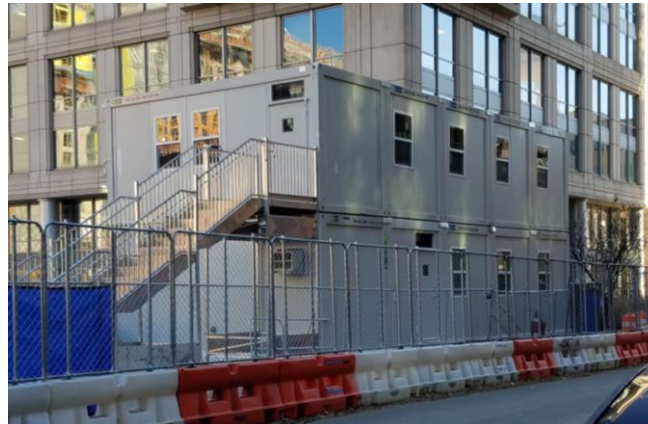
A two-story (5 over 5) FLEX building is being used by Skanska USA Building workers as office space in Washington, D.C. A 60-ton Hydraulic crane was used to set the units into place.
